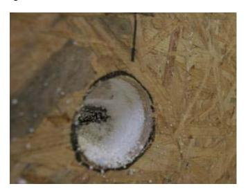
Using a spirit level, a pencil line is drawn from the new opening down to the 1200mm horizontal chasing and a second hole is cut into the OSB at that 1200mm level. The EPS must be removed to expose the factory cut chasing behind. Place a card into the lower hole to funnel the hot ball out of the panel when it has reached this location. Heat a 20mm-25mm ball bearing with a torch. You want the colour to be just under red.
